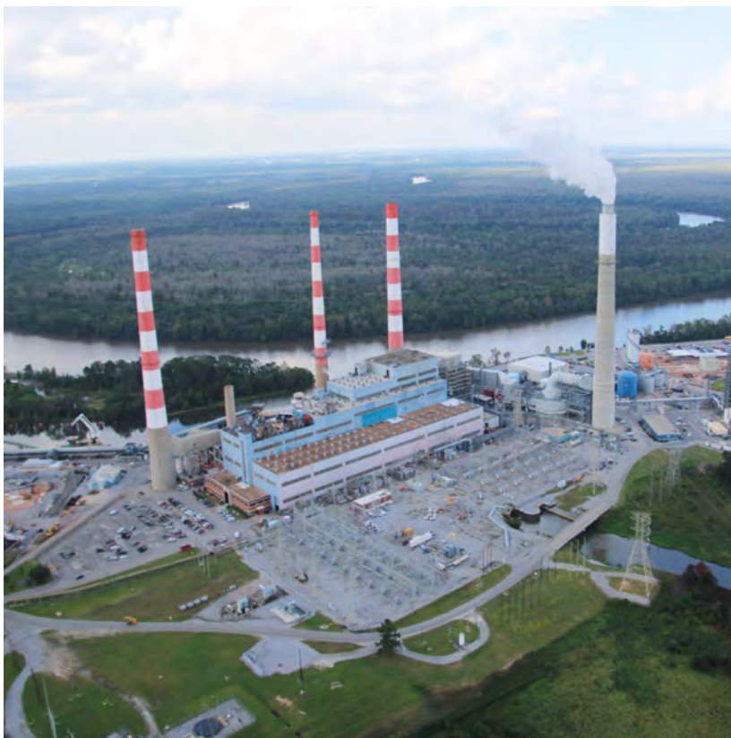
Alabama Power James M. Barry Electric Generating Plant
