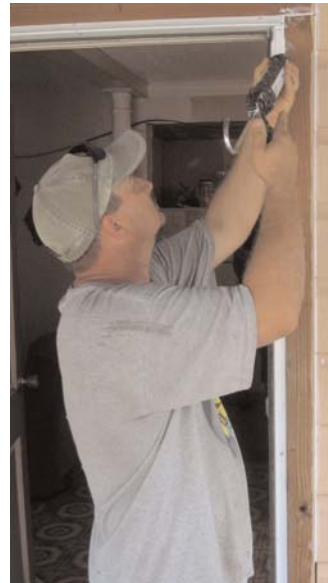
Weatherstripping around doors and windows is part of the Alabama Weatherization Assistance Program's energy audit
