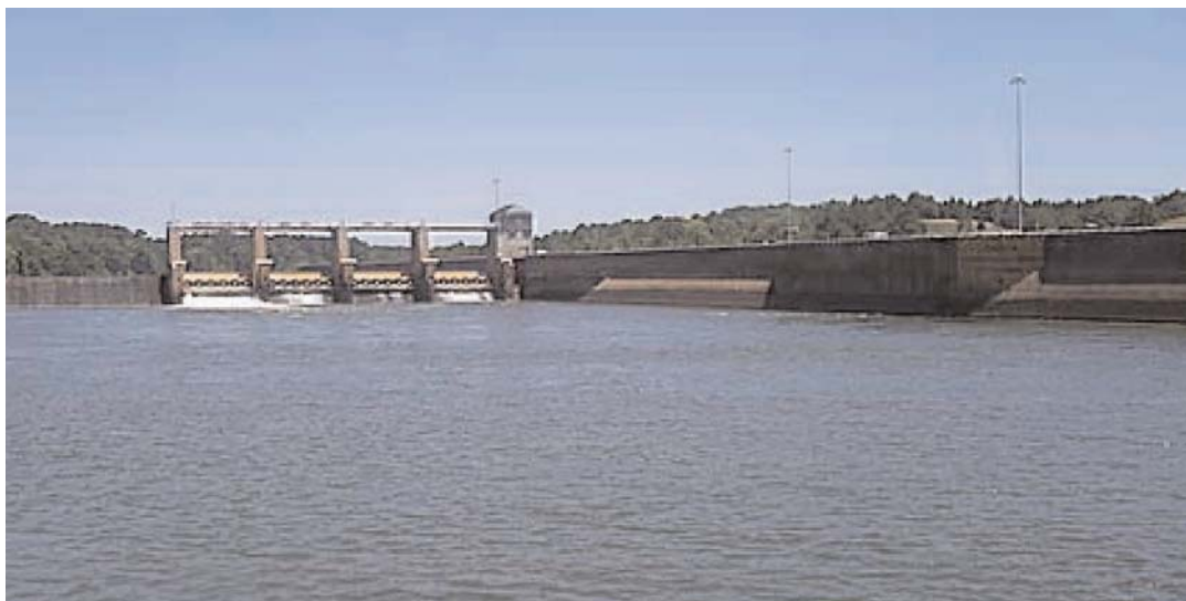
George W. Andrews Lock and Dam Hydroelectric Project
