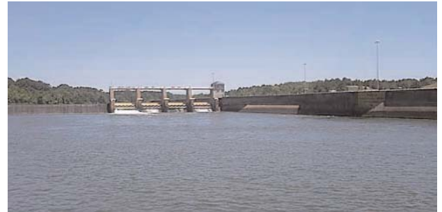
George W. Andrews Lock and Dam Hydroelectric Project
