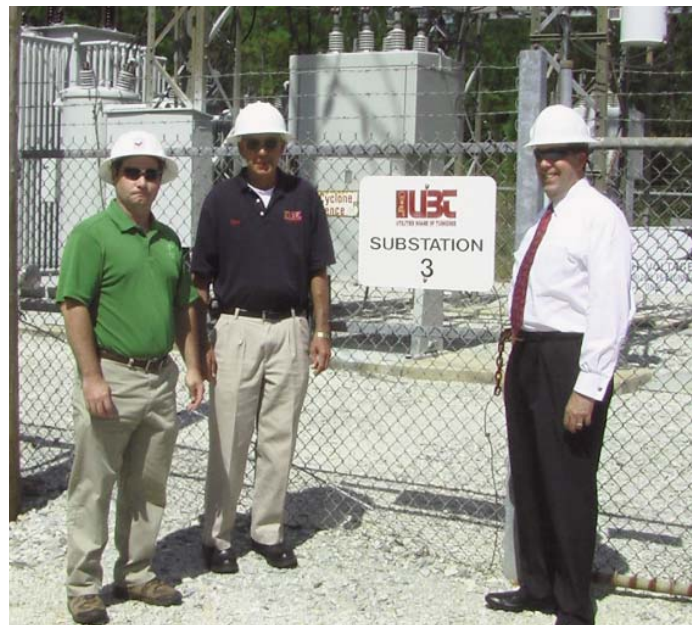
(L to R) Bishop, Posey and Harmon in a UBT substation during the AMEA Peer Review.
