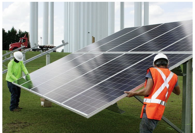
Solar panel installation in Dothan
